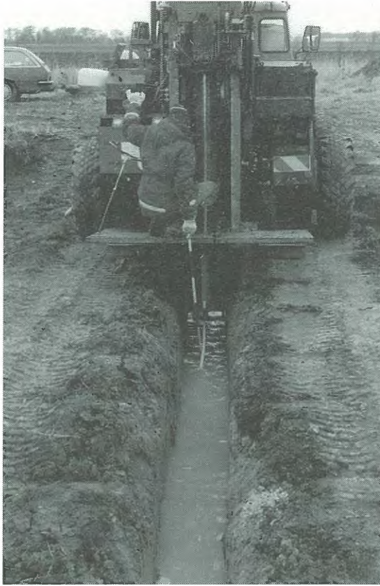
Figure 4.7 Duct installation in a trench using a drill rig.
